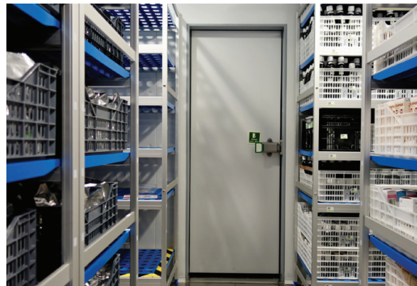
INTERIOR OF STABILCLIMA 12.000PH RUNNING AT 30°C / 75%rH
